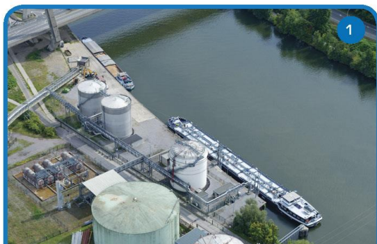
1 Riverside - Wheat unloading - ProtIWanze and Bioethanol loading.
